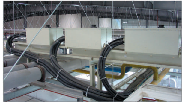
插接式母线槽Feeder busway with outlet
